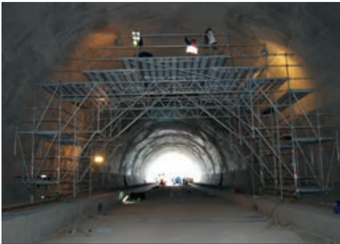
Tunnel construction in Erfurt, Germany
