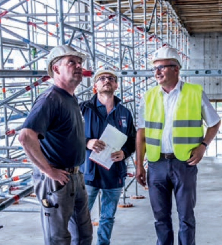
New multi-storey car park in Heilbronn, Germany
