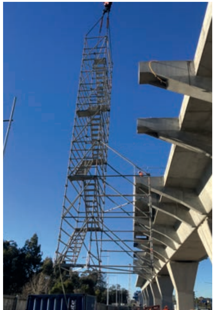
Repair of bridge in Sydney, Australia
