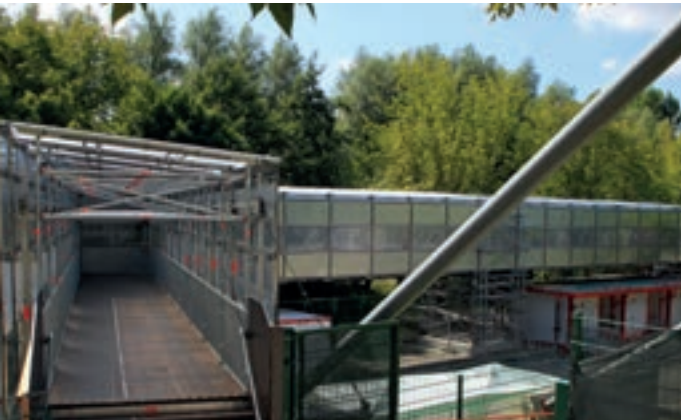
Temporary footbridge using Allround Bridging System with roofing and Protect enclosure
