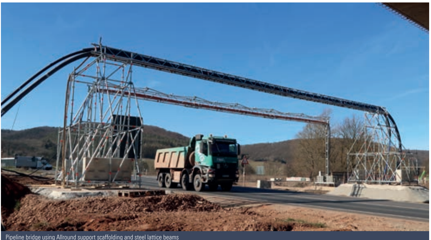
Cable and pipeline bridges made using the Allround Bridging System
