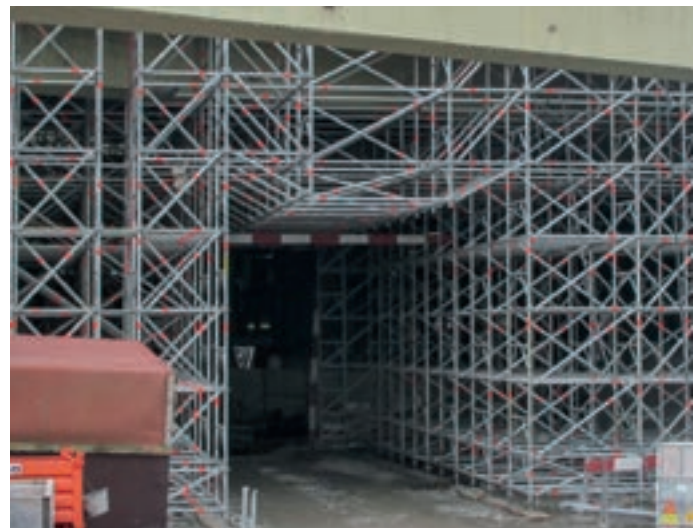
Vehicle passage opening thanks to the use of Allround standard material
