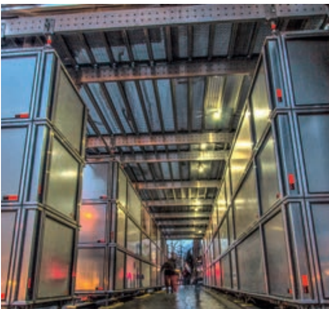
Work scaffolding with pedestrian tunnel with FlexBeam and Protect enclosure
