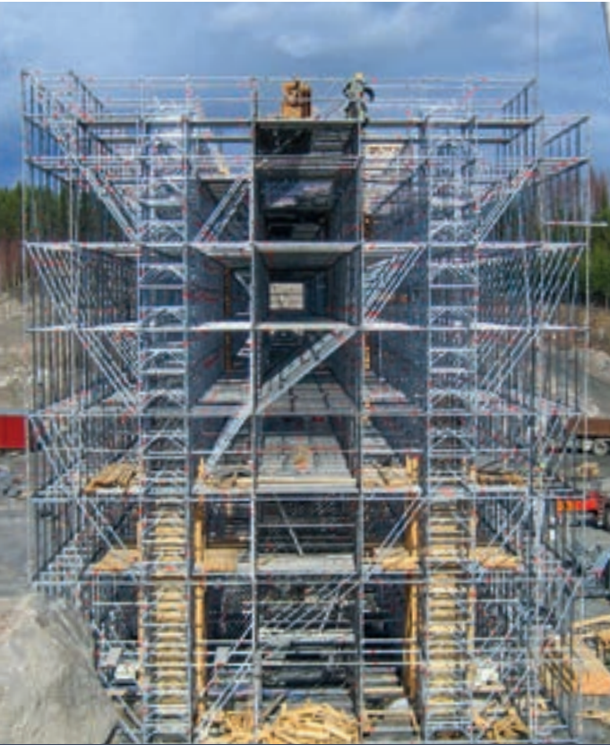
Shoring made from Allround Shoring TG 60 and Allround Scaffolding during construction of a road bridge
