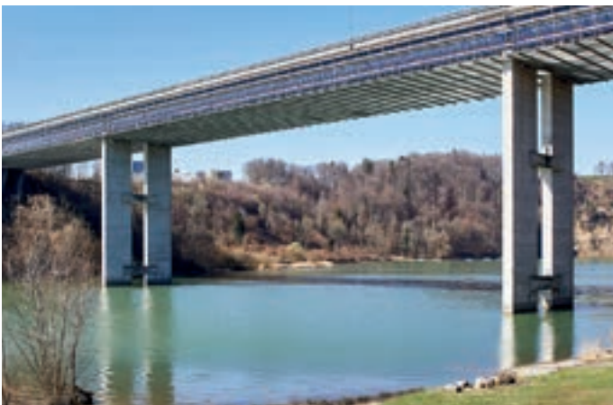
Repair of bridge in Fribourg, Switzerland
