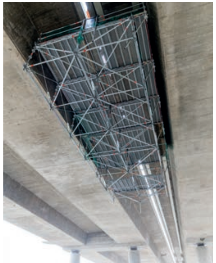
Mobile bridge underside scaffolding using Allround FW System and system decks
