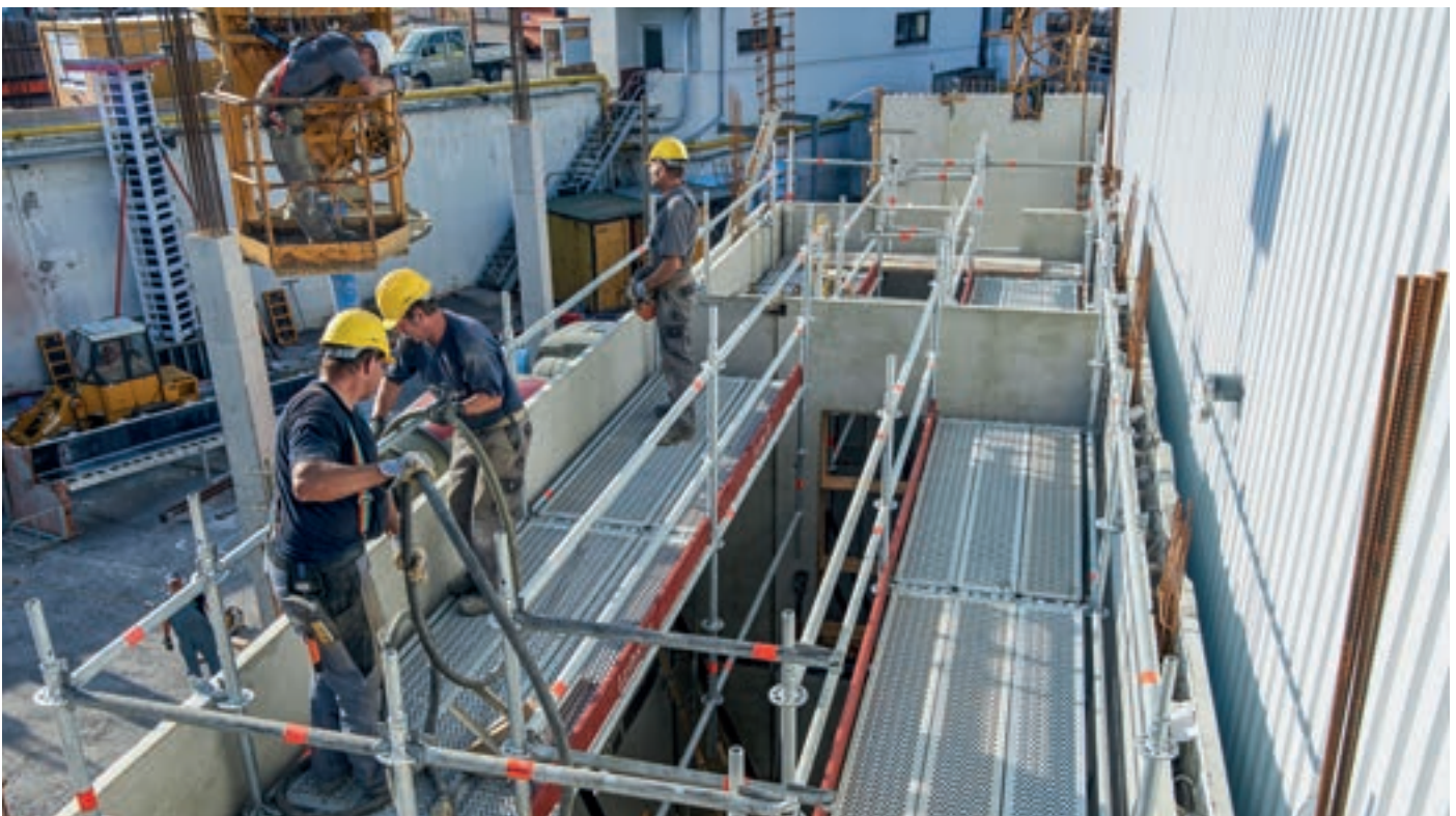
1.09 m wide concreting scaffolding with cavity wall bracket adapter
