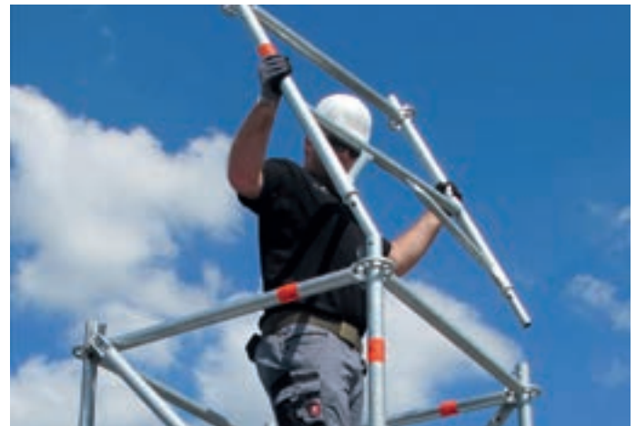
System-integrated advancing side protection during assembly of shoring towers TG 60
