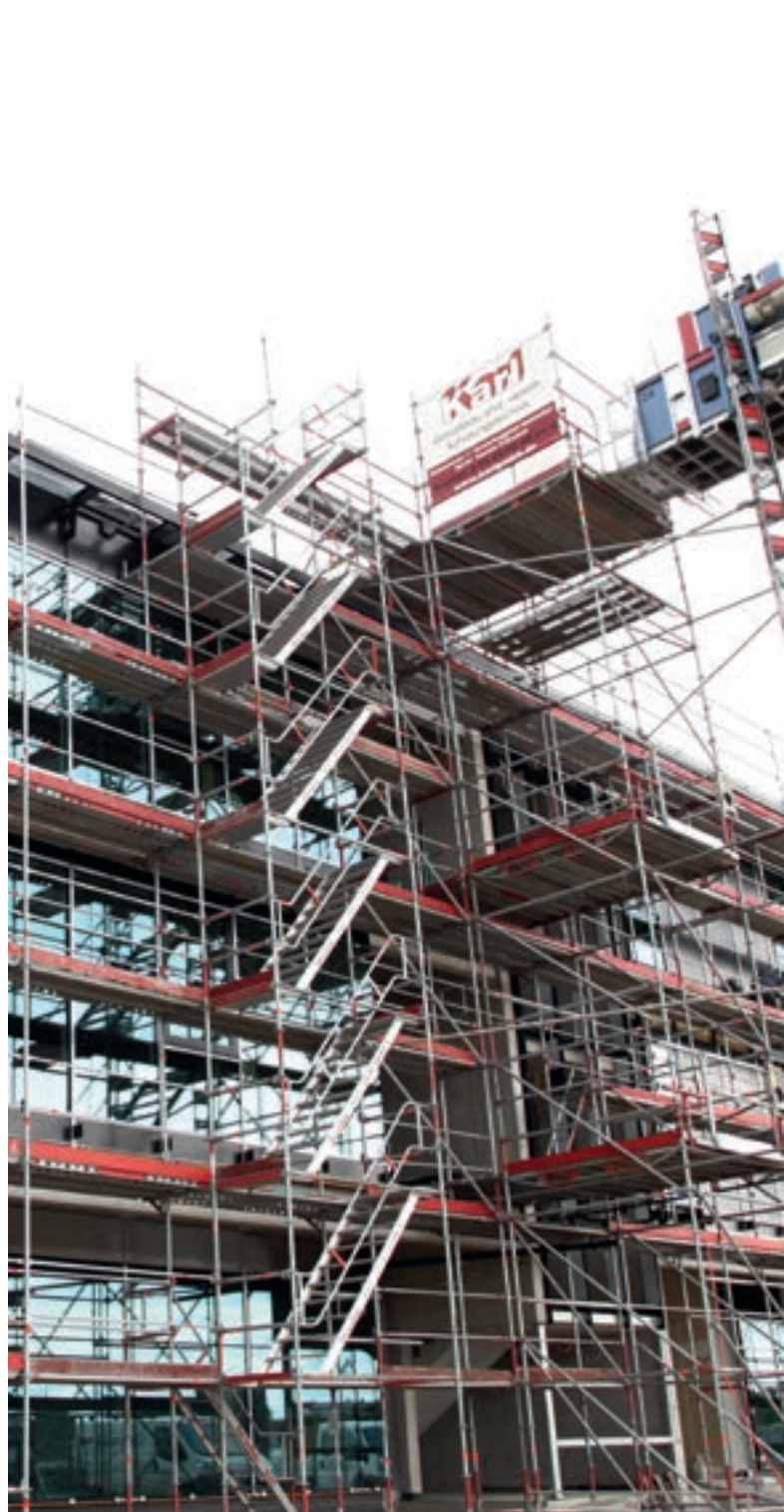
New office building in Bamberg, Germany
