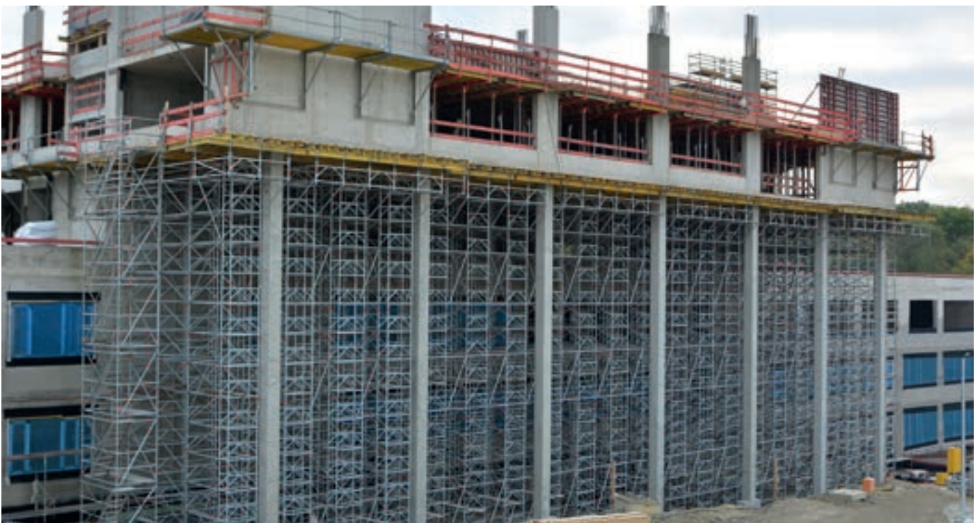
Combination of Allround Shoring Towers TG 60 for concreting of a projection — fast and convenient site access with Allround modular stairtower
