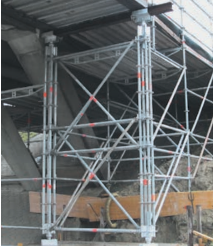
Heavy-duty support during bridge construction
