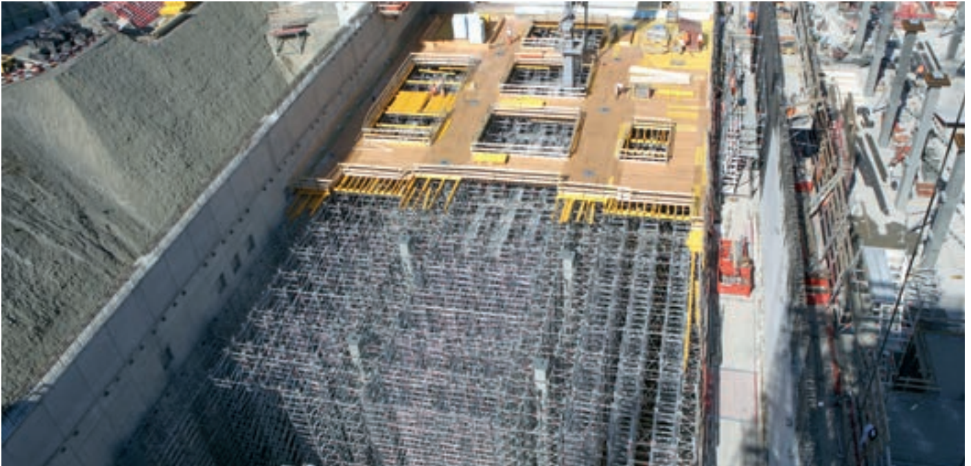
The challenge with this shoring structure was a crosswise-pretensioned slab structure for supporting a high-bay warehouse.
