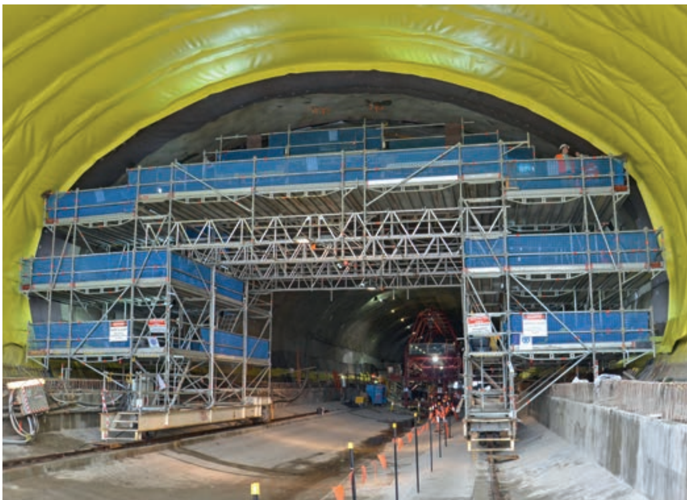
Mobile tunnel scaffolding running on rails
