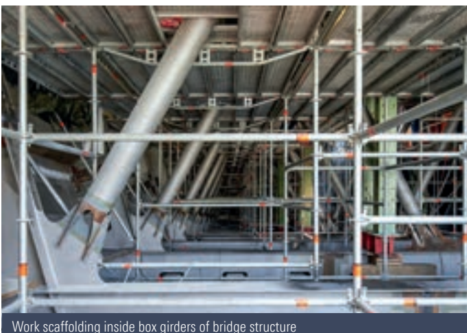
Suspended bridge underside scaffolding of lattice beams
