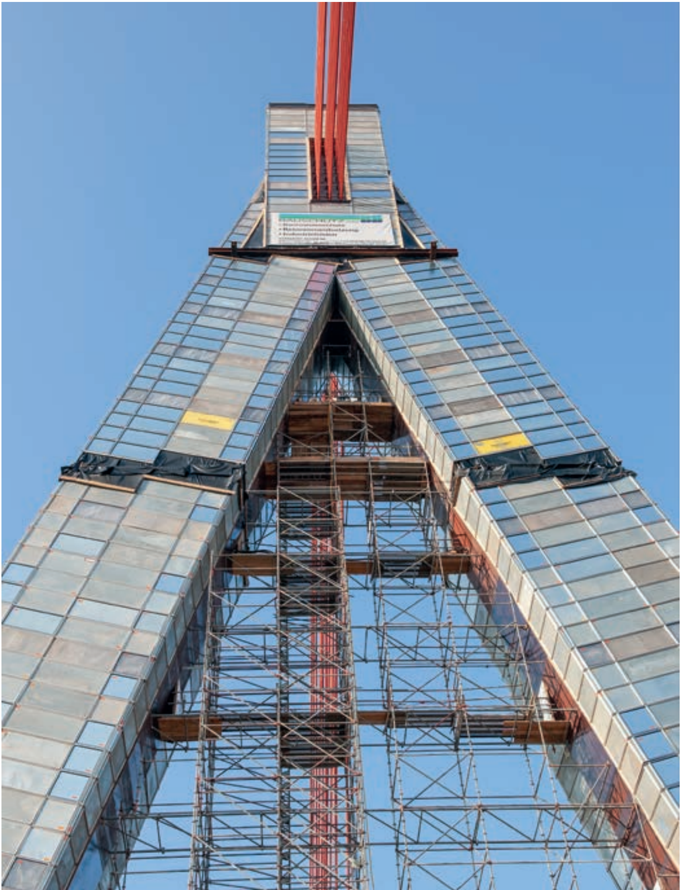
Bridge pylon enclosed using Protect System during sandblasting work
