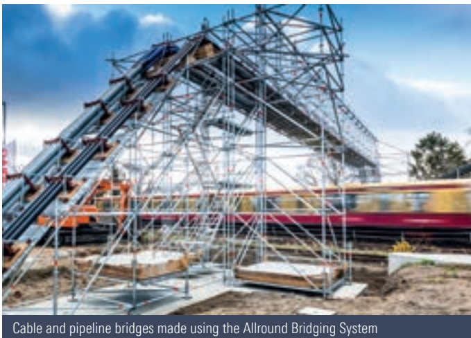
Pipeline bridge using steel trusses
