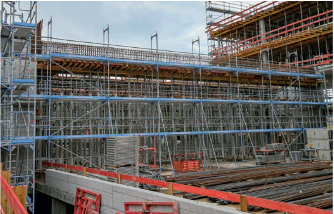
Free-standing SpeedyScaf – stability thanks to stabilisers
