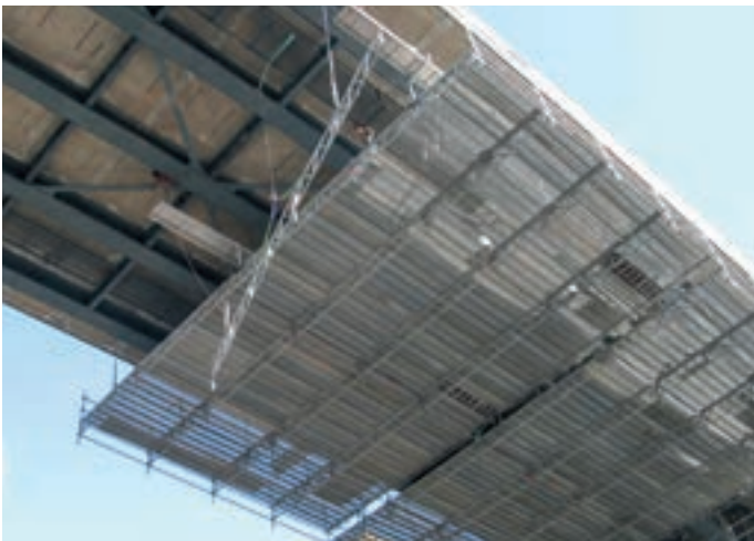
Suspended bridge underside scaffolding of lattice beams
