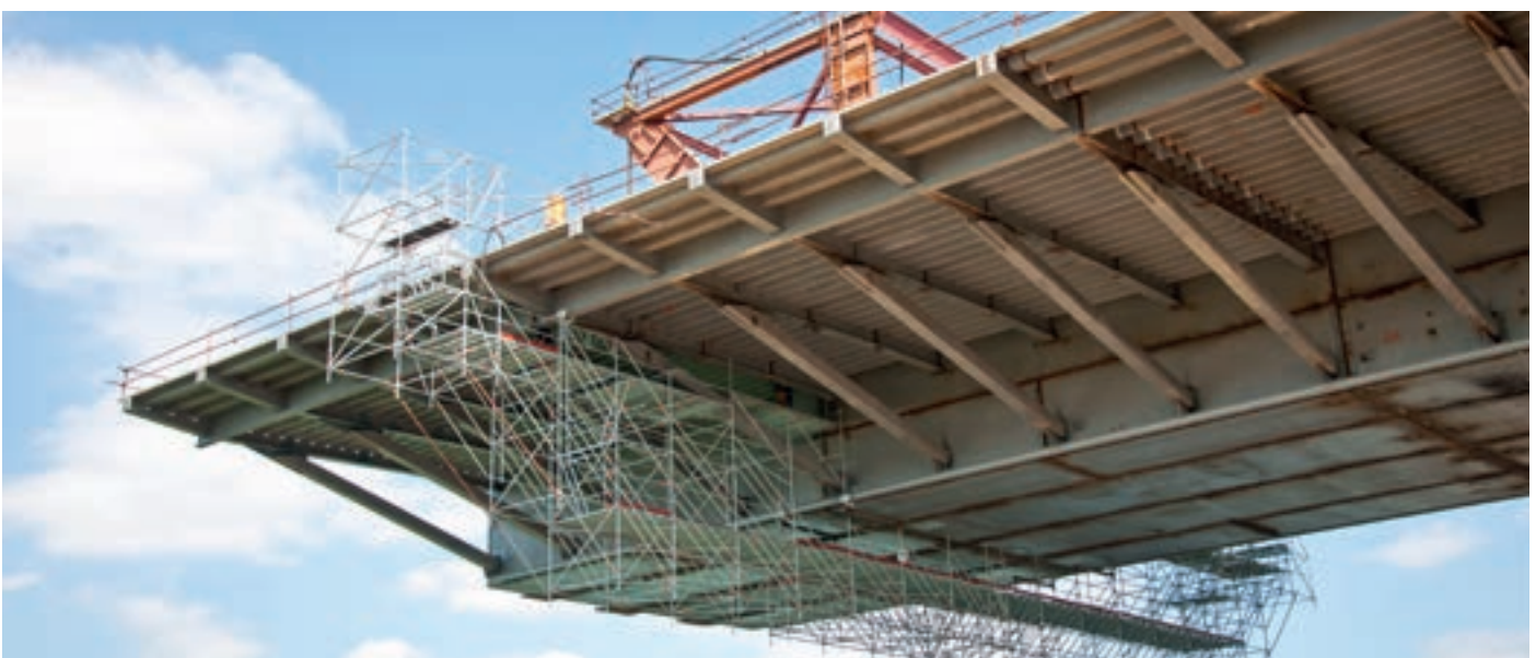
Mobile bridge underside scaffolding made of Allround system components
