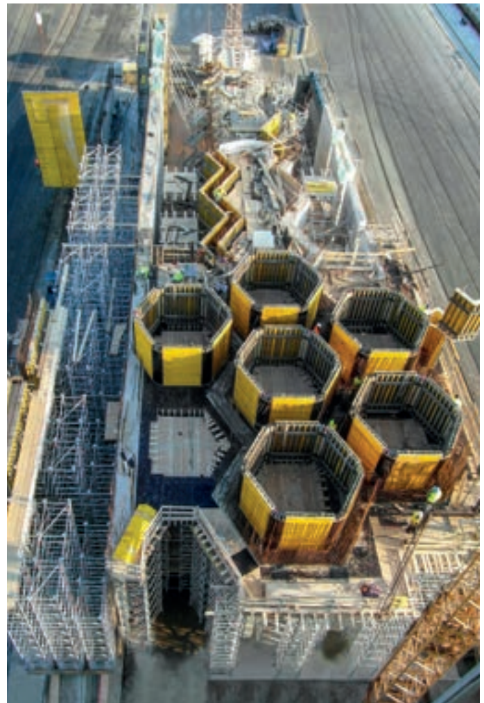
Industrial plant construction in Brake, Germany
