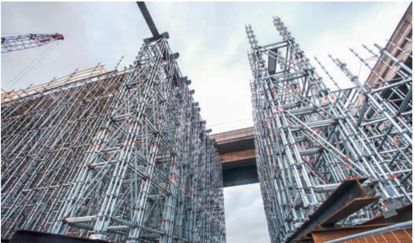
Shoring made of several combined heavy-duty columns in bridge construction
