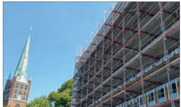
Facade work scaffolding with I-Guardrails
