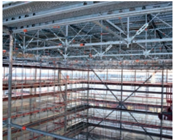
Self-supporting birdcage scaffolding in a shopping centre
