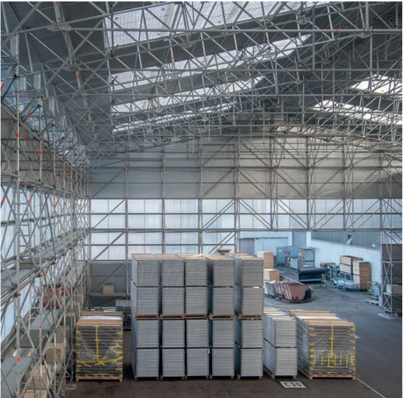
Temporary hall using Allround Scaffolding, Protect System and cassette roof
