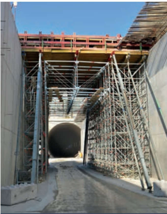
Allround Shoring Frame TG 60 with integrated FW System for vehicle passage opening
