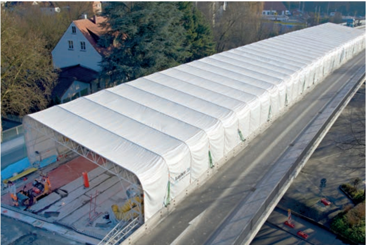
Keder Roof XL on SpeedyScaf for wintertime road construction work
