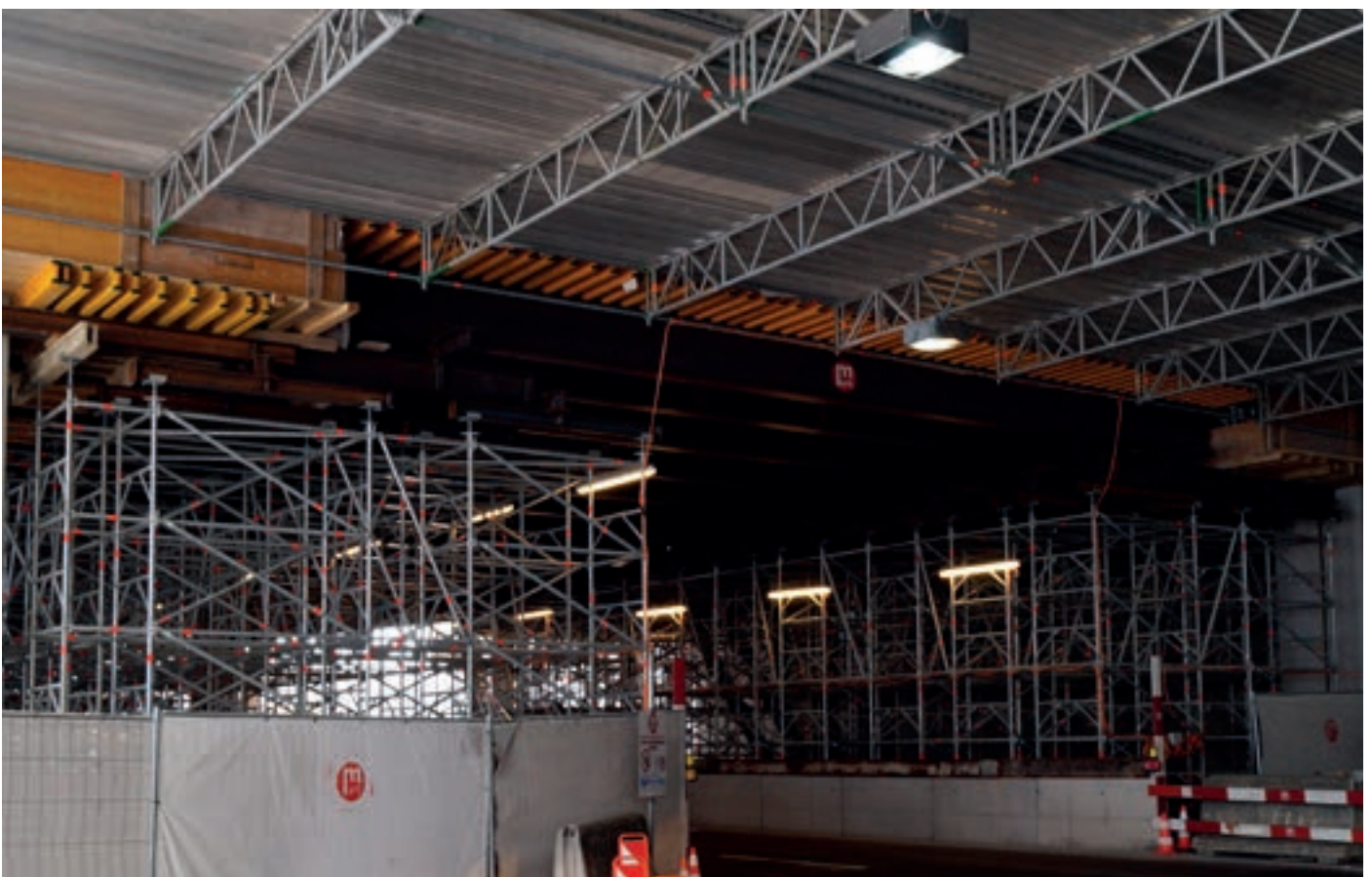
Shoring TG 60 and suspended birdcage work scaffolding made from Steel Lattice Beams 450 and system decks
