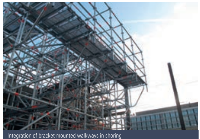
Integrated deck levels inside the shoring
