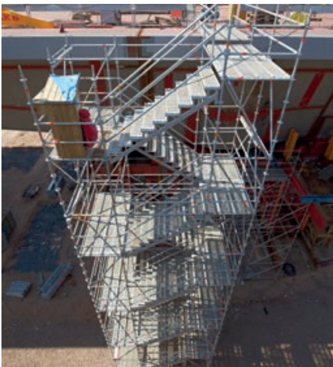
Site stairtower 200 for access to road surface
