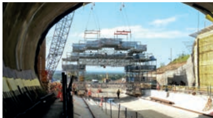
Previous emplacement of a preassembled mobile tunnel scaffolding by crane
