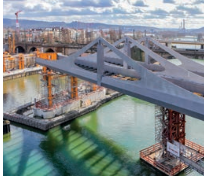
Building of new bridge in Stuttgart, Germany
