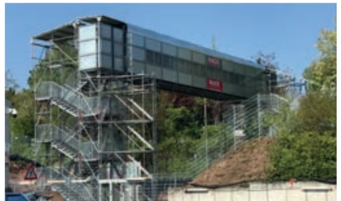
Temporary footbridge with Protect enclosure and cassette roof
