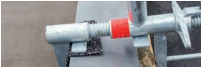
Use of a balustrade clamp on a flat roof with high fascia
