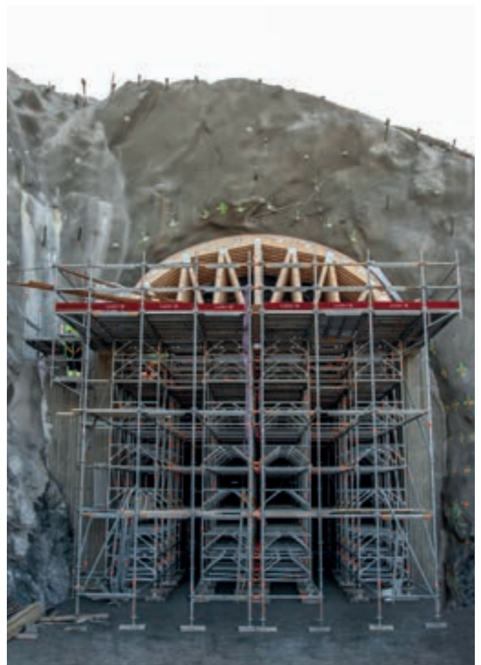
Shoring TG 60 for tunnel concreting work
