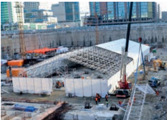
Keder Roof XL for wintertime foundation concreting work
