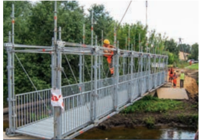
Temporary bridge with approx. 18 metre span
