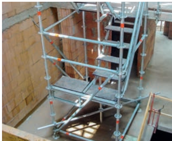
Compact stairtower in a residential block
