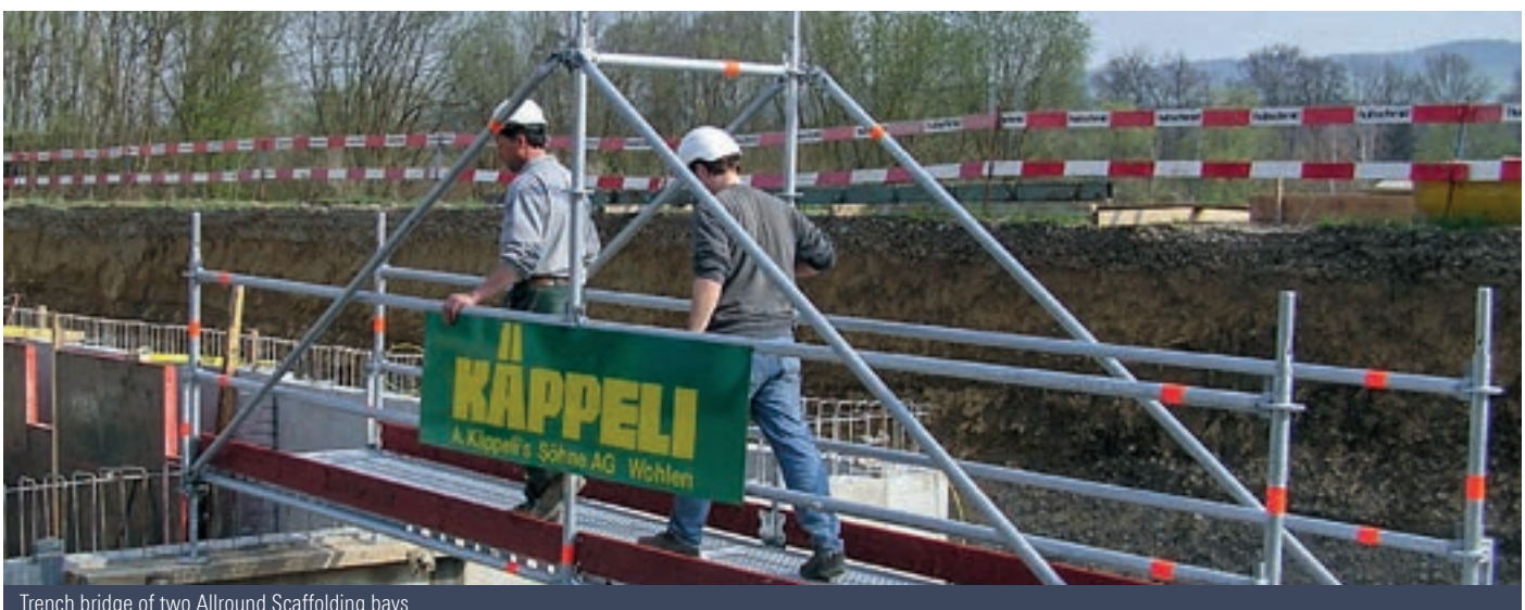
Trench bridge of two Allround Scaffolding bays
