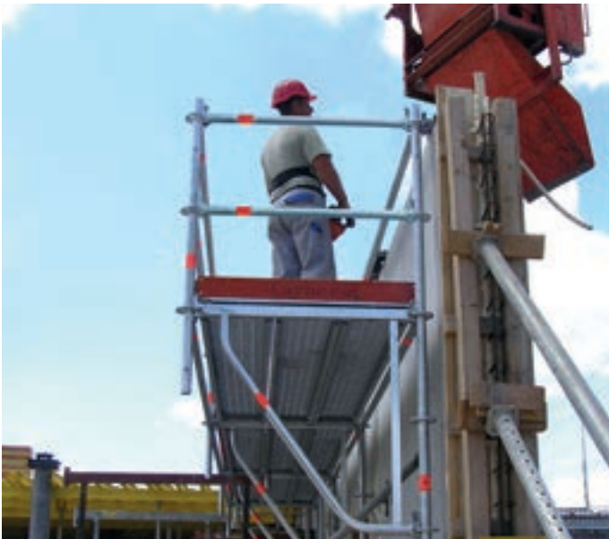
1.09 m wide concreting scaffolding with cavity wall bracket adapter
