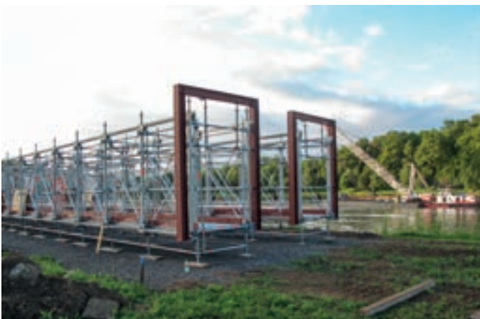
Preassembled bridges for subsequent lifting into place by crane
