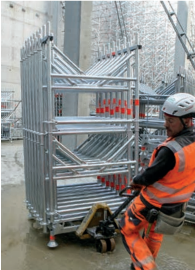
Filled TG 60 frame pallets can simply be moved on the construction site by a pallet truck.
