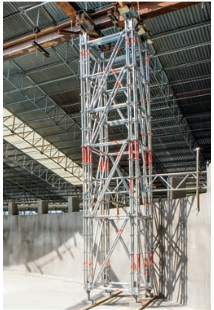
Allround heavy-duty column as a support for a temporary weather protection roof
