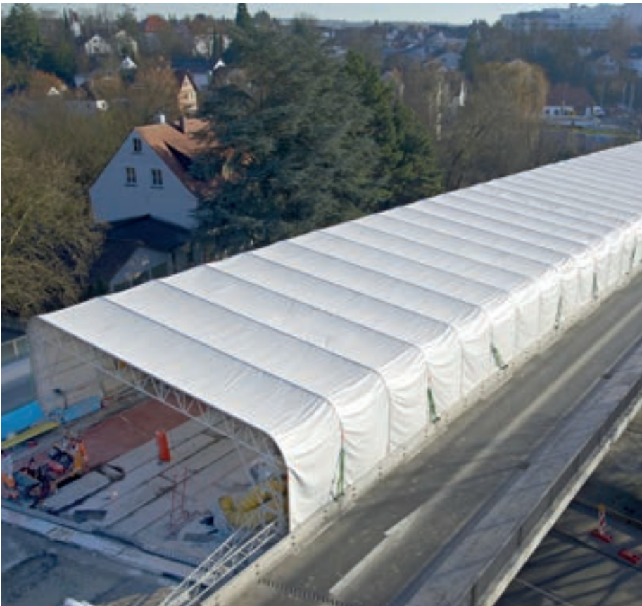
Road surface repair regardless of weather conditions
