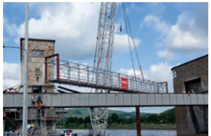
Lifting the temporary bridge into place using a floating crane
