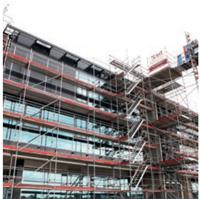
Allround work scaffolding with Allround Guardrail System
