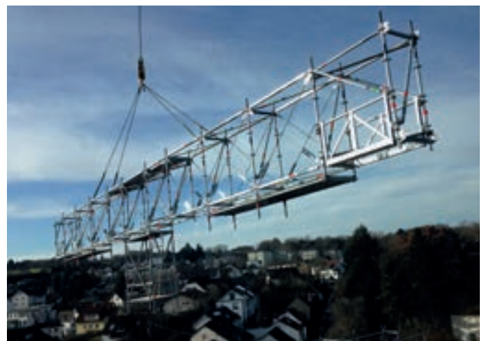
Crane movement of an FW System bridging structure
