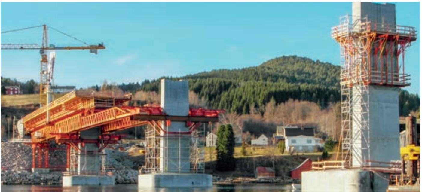
Enclosure of bridge piers as access to the formwork carriage
