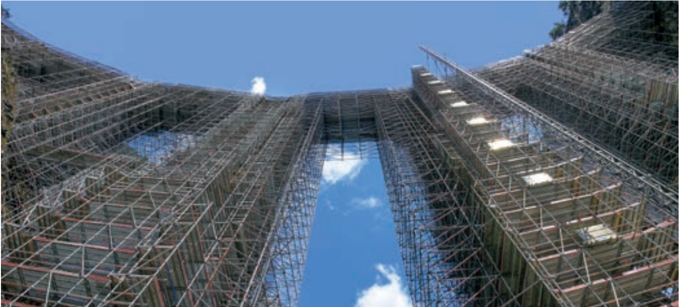
Free-standing work scaffolding on stone arched bridge
